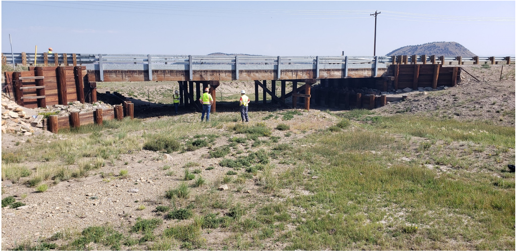
Figure C4: Ground Level Looking Downstream
